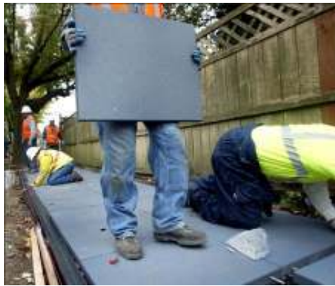
Rubbersidewalks installation
