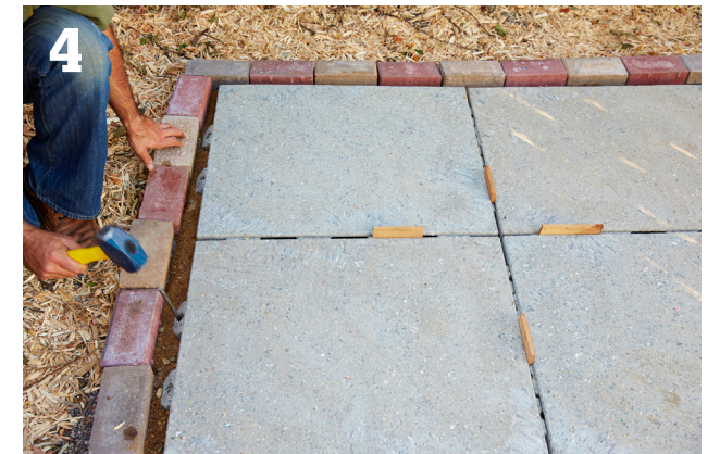
4 Pound in 10" spikes through the center tab of each paver along the perimeter of the patio. The interlocking tabs hold the other pavers. Don't use more than one spike on any single paver edge.
