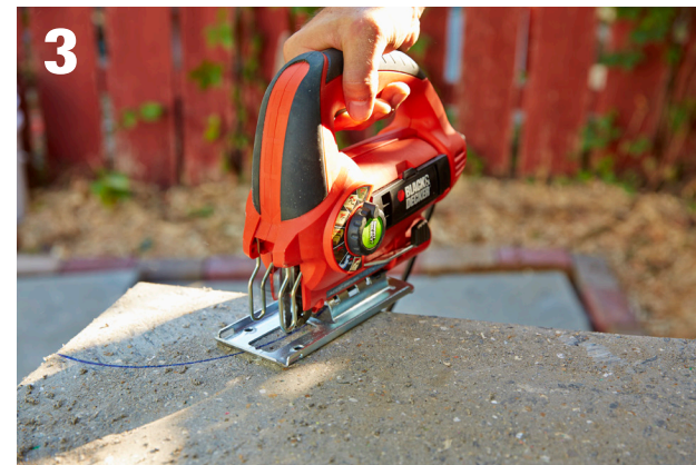
3 Make cutouts for trees or other nonsquare items using a jigsaw. Use a circular saw guided by a straightedge to make straight cuts in the pavers. Don't be tempted to cut off the tabs around the outside edge—they help anchor the pavers and should be left in place.
