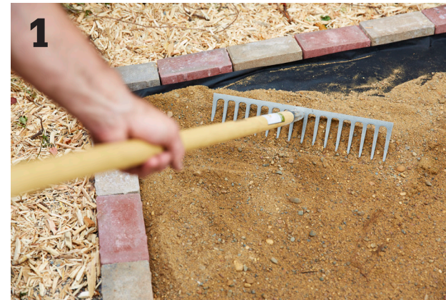
1 Prepare the subsurface by digging down enough for a minimum of 2" of ¾" angular gravel plus a setting bed and allowing for the thickness of the pavers. Soak and compact the gravel, then add sand, and screed the surface smooth and level. See pages 122 to 125 for more information on preparing a permeable base.
