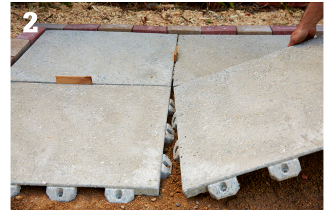
2 Tip the pavers in place so the tabs connect as you lower the pieces. Use ¼" spacers in the joints for a clean look and to assure drainage. Keep the spacers in place until all pavers are installed. Do your best to level each paver as you set it in place.
