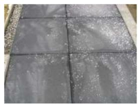
The photo to the left depicts the Rubbersidewalks™ installation at the Unalaska Community Center. It is the most extreme example of a cold weather installation. After almost five years, the application is highly successful and has no damage as a result of the use of both Ice Melt and rock salt. The photo to the right is a close up shot.
