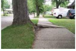
"A pilot study done by City Engineer, Boyd Phelps documents that it cost the City only \$367 more to install Rubbersidewalks instead of pouring back concrete to save 2 Pin Oaks. The Oak trees were valued by a Purdue University formula at \$8,580 and \$11,206."
